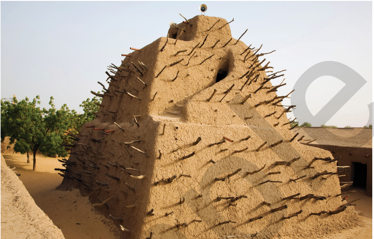
This pyramid structure, built in 1495 CE, marks the tomb of Askia Muhammad. It stands in the city of Gao and is located between two mosques. Similar to most West African buildings, it was constructed using mud brick reinforced with wood.
